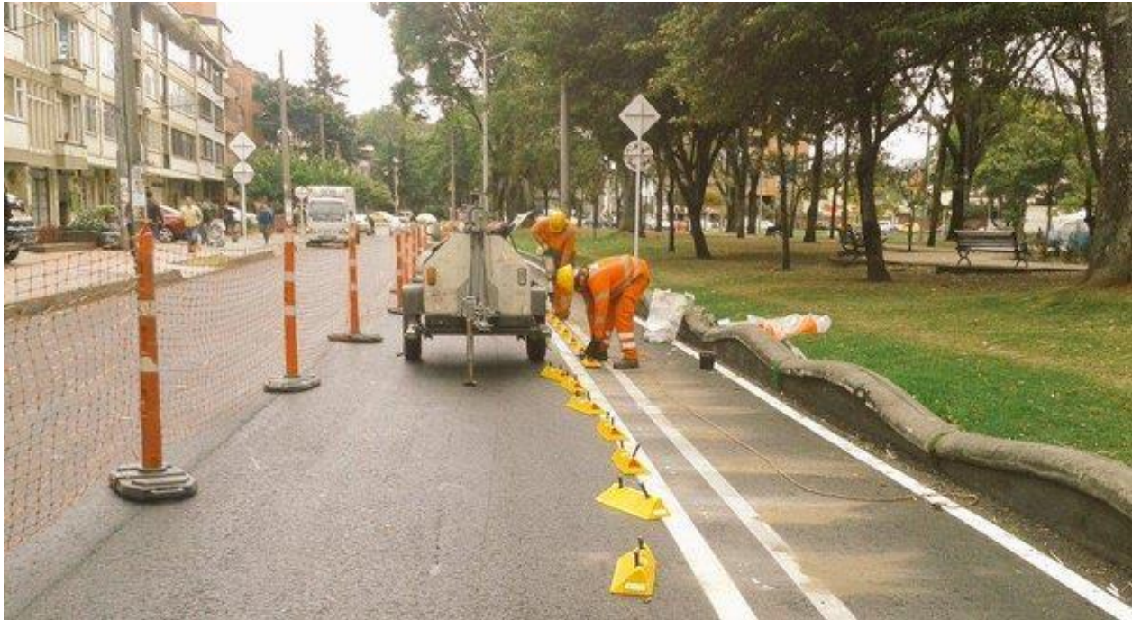
Fig. 6. Employees from IDU making the pilot project of Teusacatubici permanent (IDU Bogotá, 2015)
